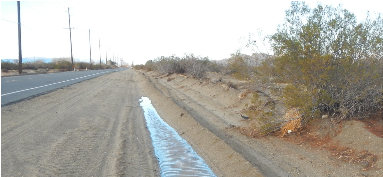
Figure 2. Standing water in a ditch near Lake Los Angeles following rain. Creosote is growing vigorously on the elevated ridge constructed when the road was built.
