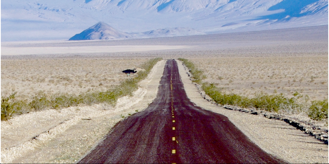
Figure 1. Enhanced Creosote growth on the elevated ridges on either side of Trona Wildrose Road in Panamint Valley. Note the more widely spaced and smaller creosote bushes in the undisturbed soil well away from the road.
